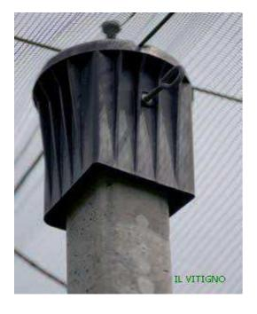
The covering caps are placed with pressure on the upper end of the pole, which fit perfectly without coming off since the section of the hole is slightly smaller than the pole. As a further precaution it has been used an eye screw to fix the cap permanently. The poles covering caps serve for the fixing of longitudinal and transversal wires and ropes; furthermore they are required to protect the mesh or the plastic film from possible damages caused by the rough surface of poles.
